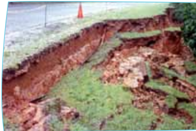
Palau National Weather Service Office
