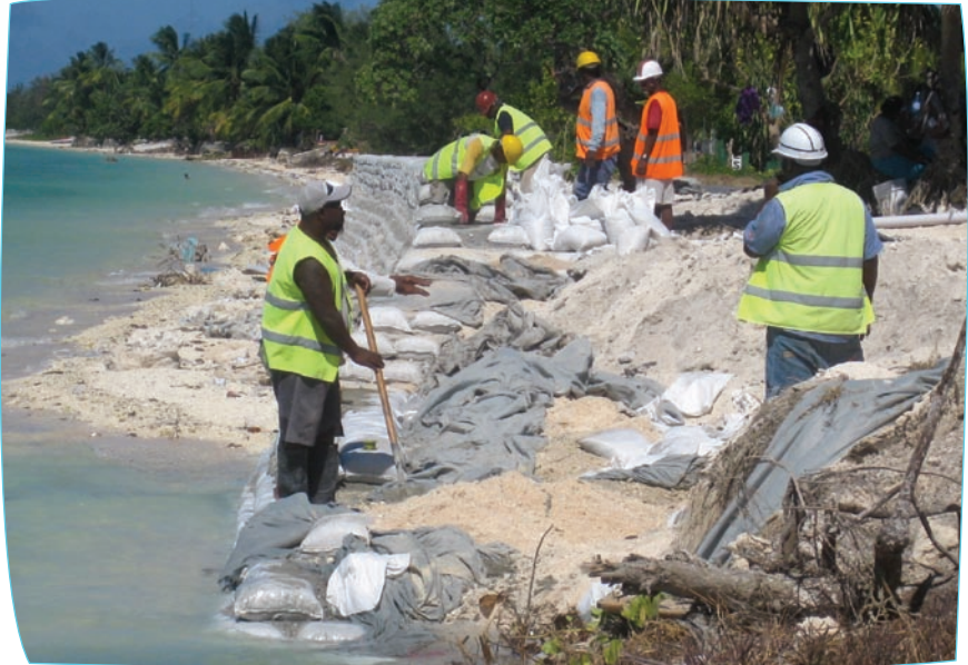
Sea defences under construction in Kiribati
